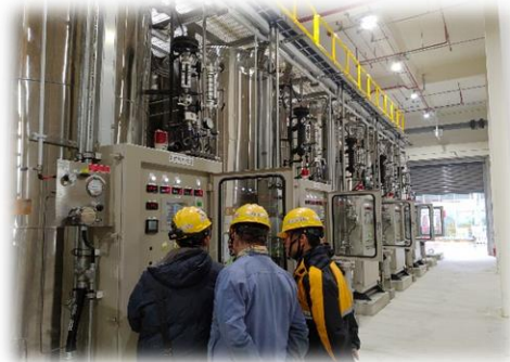
燃氣鍋爐設置
