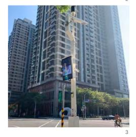
1. New Taipei is upgrading to smart LED streetlights to enhance lighting quality and energy efficiency. 2. Smart streetlights detect issues and report them instantly, speeding up repairs and improving nighttime safety. 3. The city pioneered Taiwan's "pre-embedded shared pole" system, installing smart pole foundations during road construction to avoid re-excavation and lower costs.
